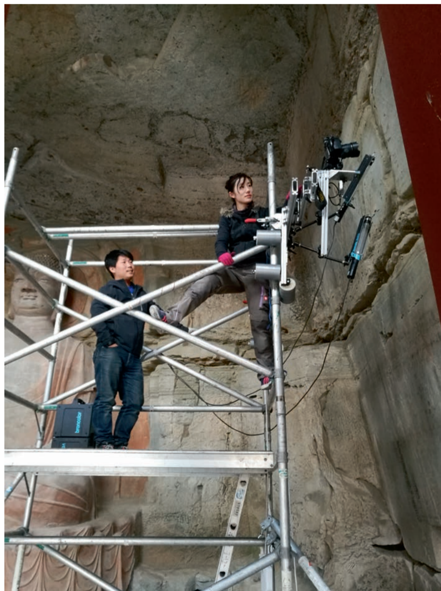
Second-generation scaffold in the cave at Jinchuanwan; photograph taken in 2017
